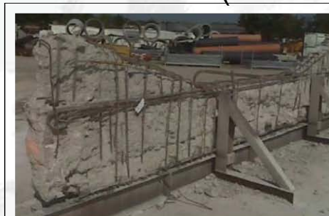
Beam after hydrodemolition
