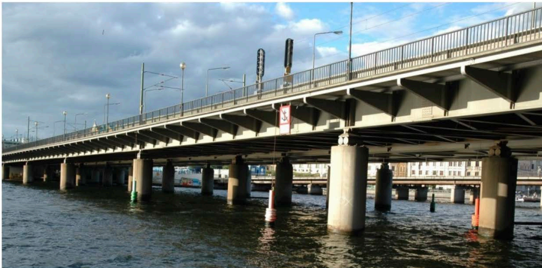
Figure 1a: A photo of the Söderström Bridge
