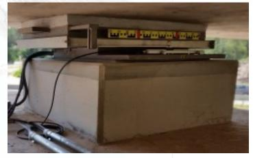
Instrumented bearing (source: BASt)
