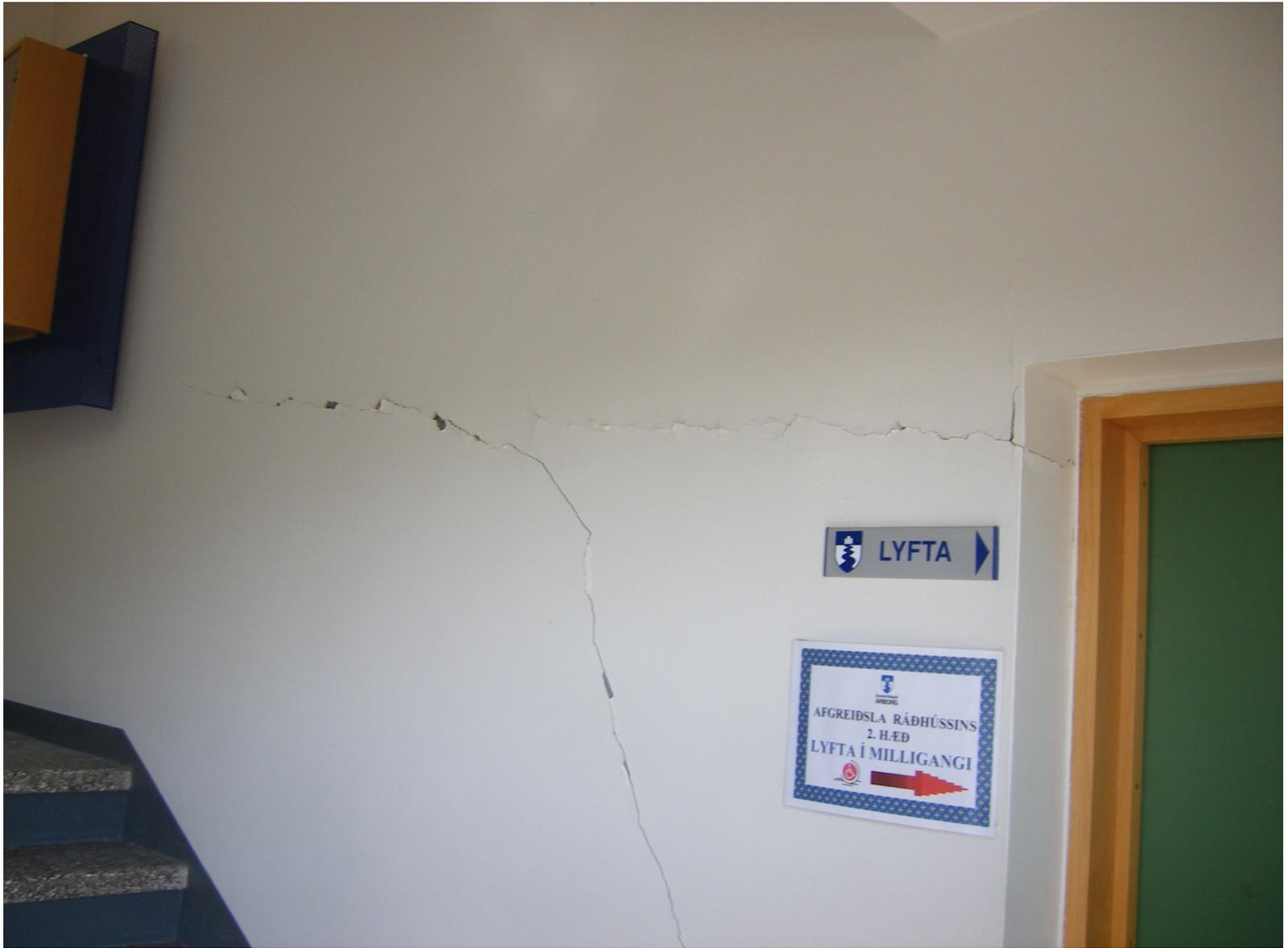
Fracturing of the stairwell shear core walls
