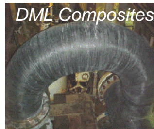
ISO/TS 24817:2006: Petroleum, petrochemical and natural gas industries -- Composite repairs for pipework -- Qualification and design, installation, testing and inspection
