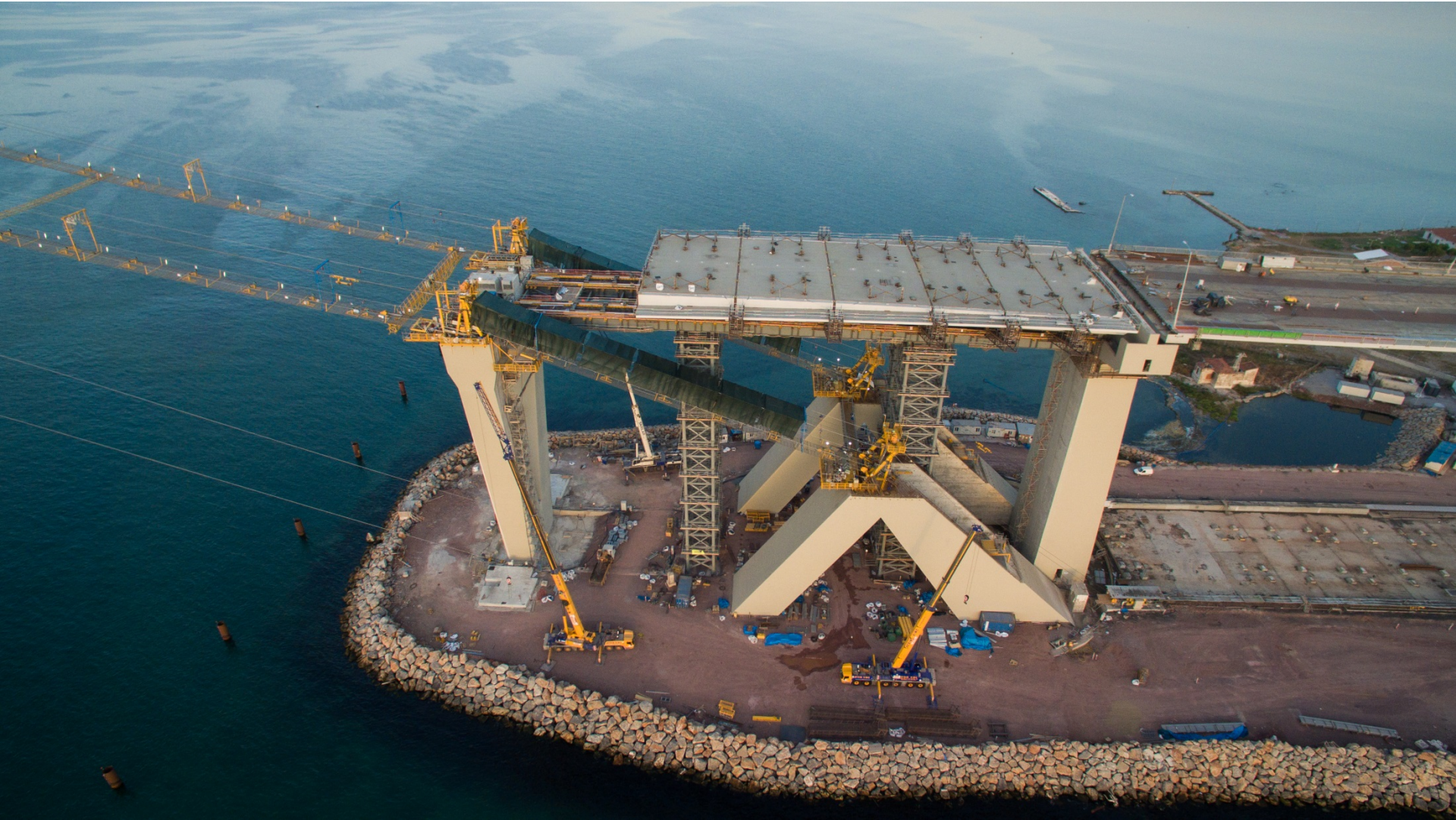
Transition Span – Deck Erection South (TS08~TS03) ACTUAL FINISH: 18-JULY-2015
