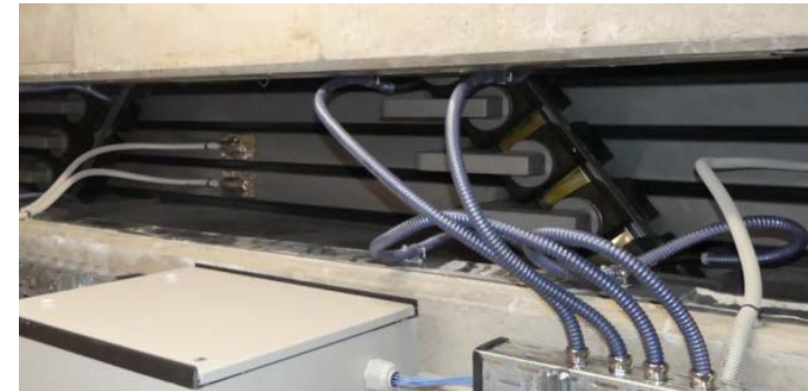
instrumented expansion joints
