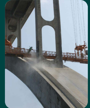
Krk: optical sensors embedded into columns
