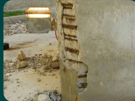
Maslenica: Reinforcement corrosion on column S10
