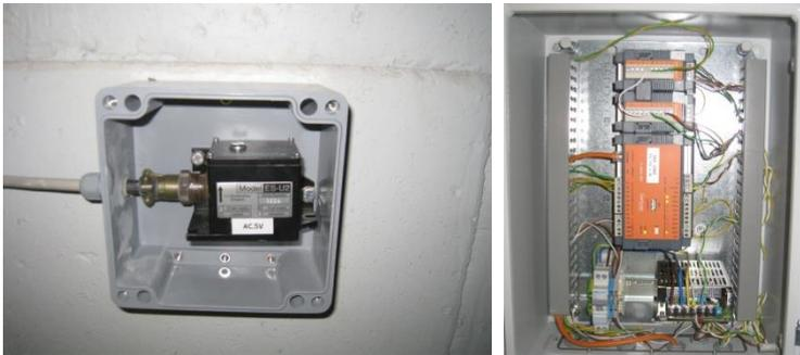
Figure 6: Structural dynamic monitoring: accelerometer and data acquisition system
