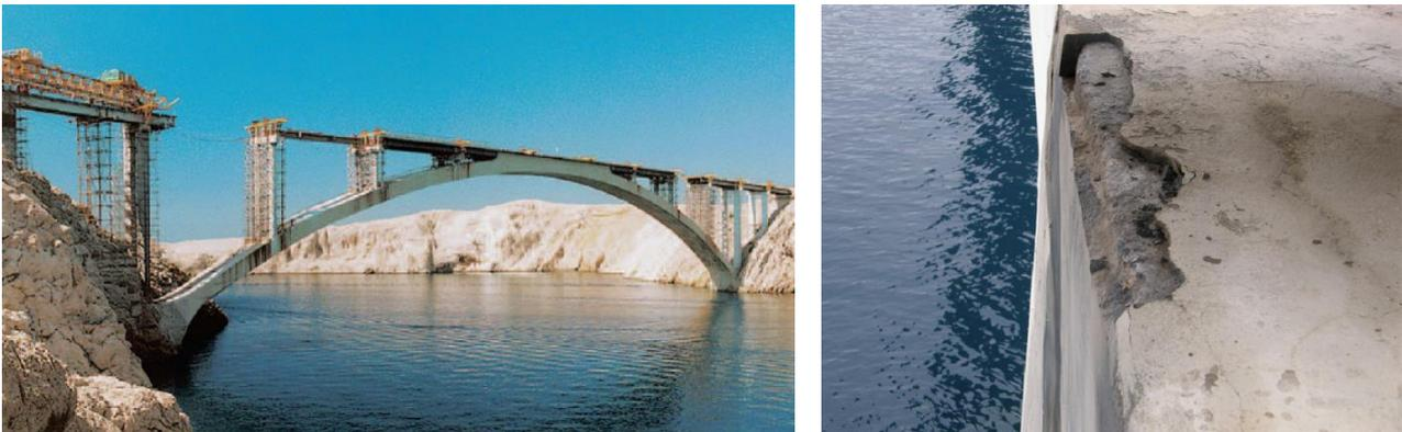
Figure 4: Pag bridge originally built in 1968 was repaired in 1999: new steel superstructure was installed by launching truss (left); delamination at the edge of the arch abutment as an example of defects in rc arch protection system (right, Bleiziffer et al. 2011)
