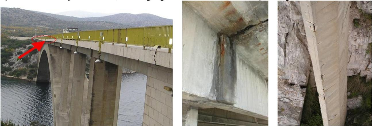
Figure 3: Deflected vertical alignment of the Šibenik bridge built in 1966 (left) and deterioration of the superstructure (middle) and columns (right)
