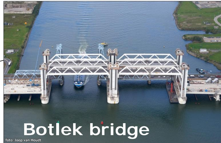
The current Botlek Bridge (combined railway and motorway bridge) will be replaced by a new lifting bridge across the Oude Maas, eliminating a major shipping bottleneck in the region. The new Botlek Bridge features two bridge passages – each around 90 metres wide – and will rise some 14 metres above water level. When completed, the new Botlek Bridge, which lifts to a maximum height of 45 metres, will be one of the largest moveable bridges in the world.
