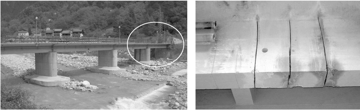
Figure 9: General view of Dogna Bridge (left, tested span circled) and detail of damages D1-D6 (right).
