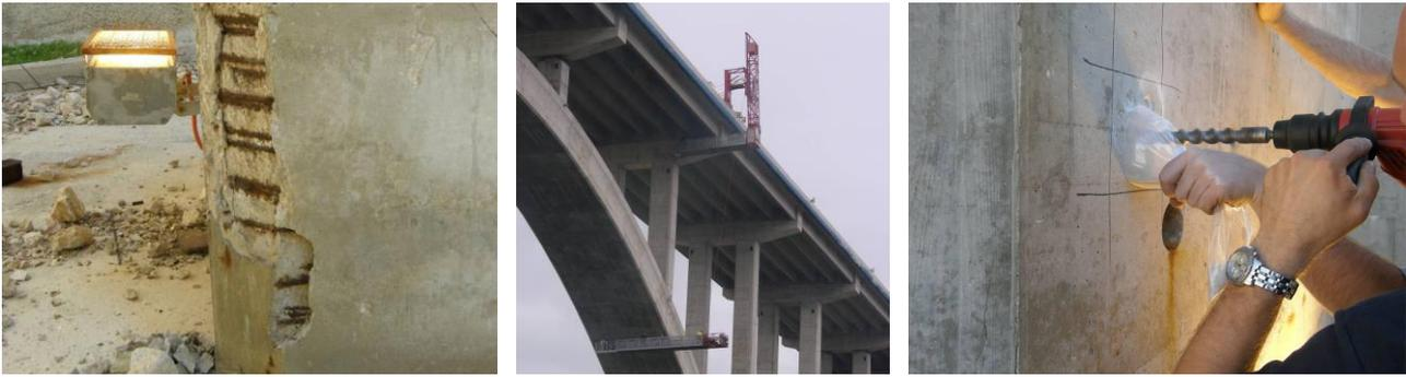
Figure 6: Maslenica bridge (Bleiziffer et al.2011): reinforcement corrosion on column S10 (Left); under bridge inspection unit (middle); taking dust samples for determination of chloride content and depth of chloride penetration into the concrete (right)
