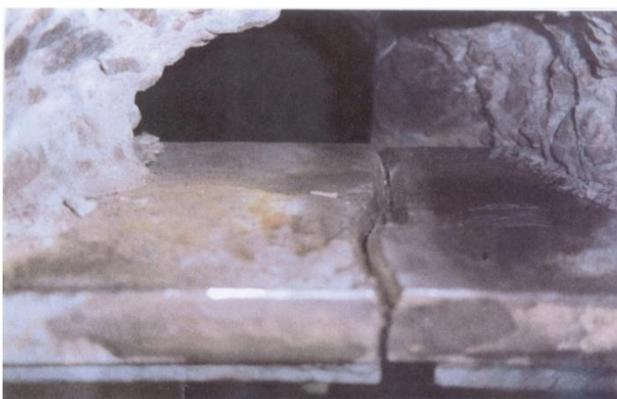
(a) The top flange of a main beam cracked through the whole width.
