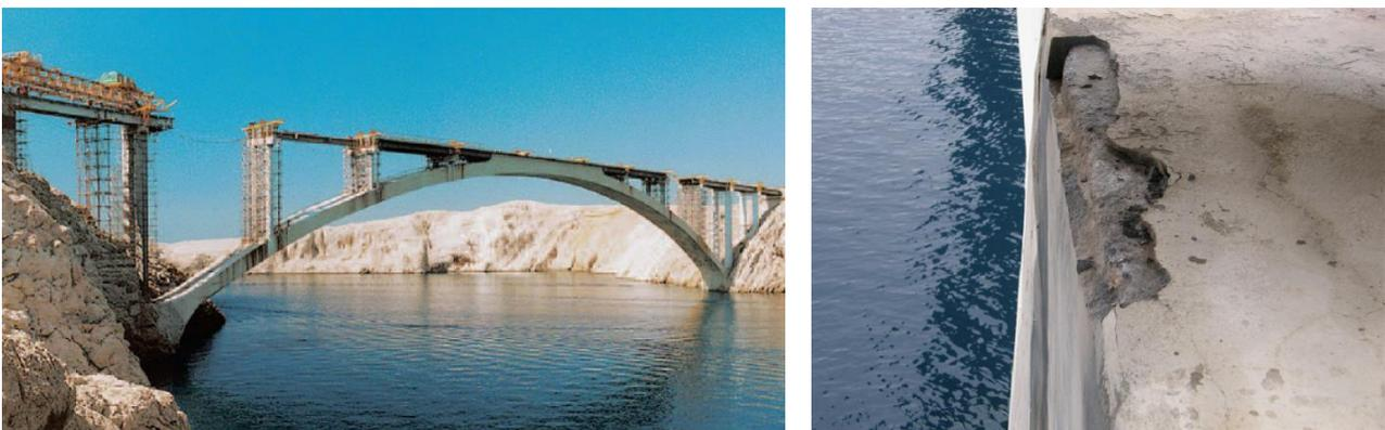
Figure 4: Pag bridge originally built in 1968 was repaired in 1999: new steel superstructure was installed by launching truss (left); delamination at the edge of the arch abutment as an example of defects in rc arch protection system (right, Bleiziffer et al. 2011)
