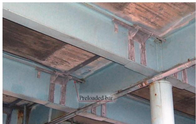
(b) Safety measures to prevent collapse in case of a propagating crack.
