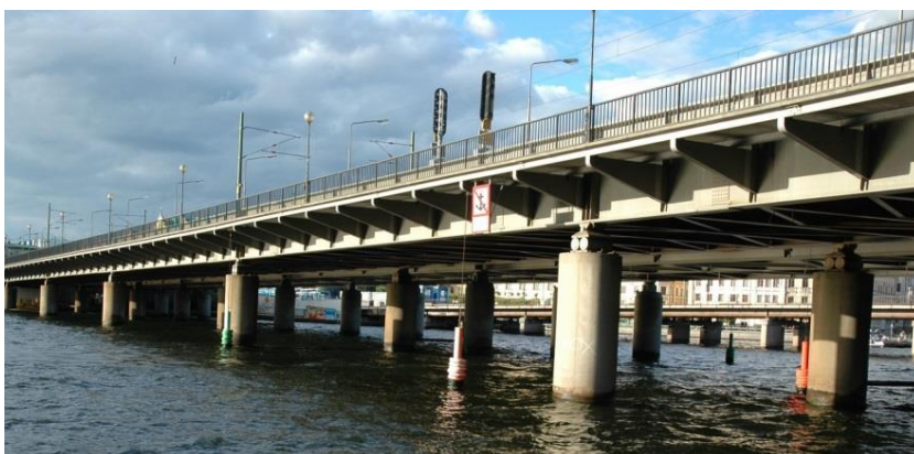
Figure 1a: A photo of the Söderström Bridge
