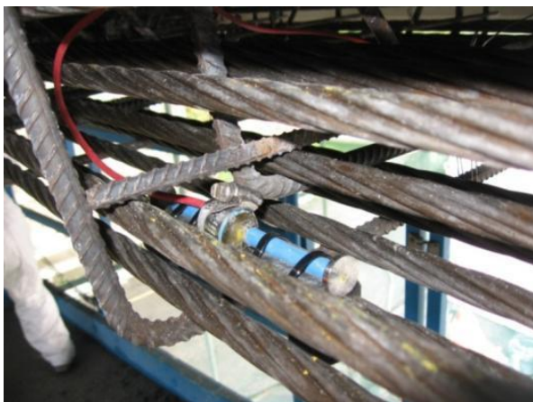
Figure 4: Installation of gauges to prestressed tendons following hydrodemolition.
