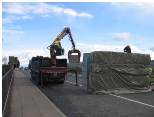
Figure 5: Removal of preload following hardening of repair material.
