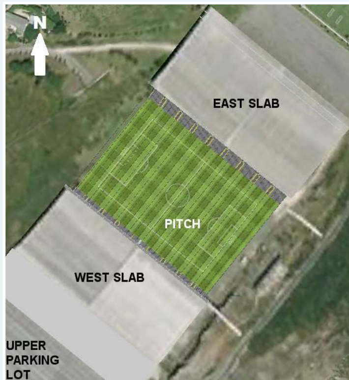
Top view of the stadium
